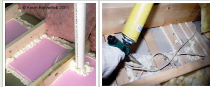
Examples of attic air sealing
